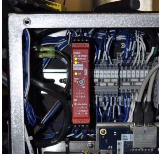
FIGURE 4-25. SAFETY RELAY LED'S
