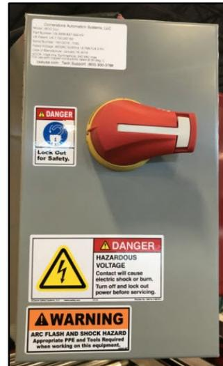
**Figure 57 – IBOD Knob Power Control Box**
